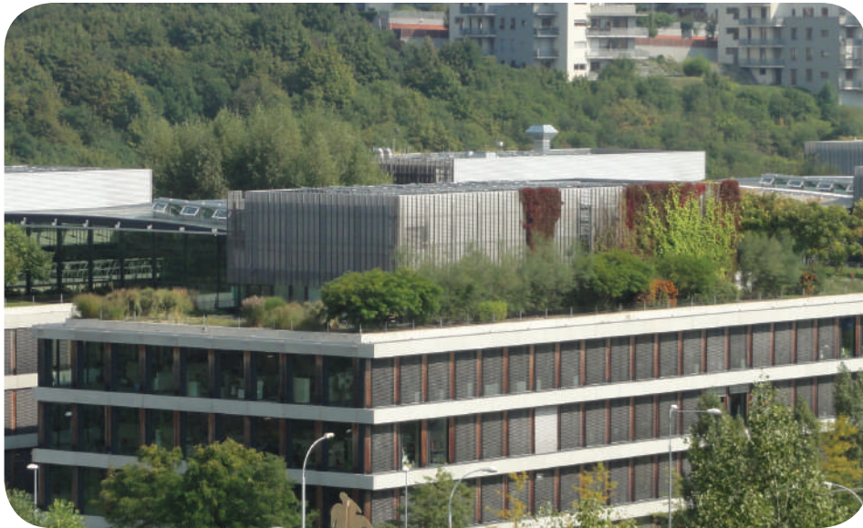
Fig. 25: An intensive green roof, vegetation shading and other energy saving measures on the ČSOB Bank headquarters in Radlická Street / Source: http://www.csob.cz
