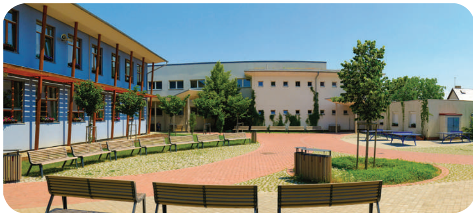
Fig. 26: Passive and low-powered Primary School and Kindergarten with an extensive green roof and a semi-permeable paving in Prague – Slivenec / Source: skolaslivenec.cz
